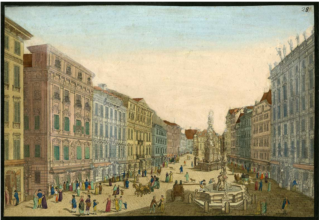
View of the relatively uncrowded Graben in Vienna around 1800.
